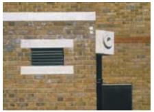
When unavoidably interior to the walls, JOA gutters are always fitted with prominent overflow outlets. This was a rainwater hopper, and overflow, in ballidon limestone concrete, to the transformer building.
