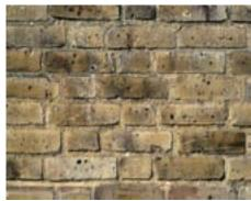
Old brickwork laid in lime mortar has small pieces of grit in its wide joints. There is none of the dead grey of Portland cement. The depth of the mortar joint is gentle - outlining the separate bricks while preserving the wholeness of the wall as a great sheet.
