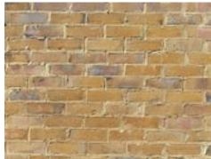
At Poyle the excess mortar 'fat' was cut off, flush to the bricks, with a single upward strike of the trowel. The joints were not 'struck' that is pushed in to solidify their surface as such a protection of the joint betrays an ignorance of how stock bricks suck rainwater OUT of joints.
