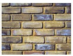
In Kensal Road the mortar was 'pointed' by being scraped back 5 mm with an American hand-held wheeled trowel. Some suppose this endangers bricks to frost attack - again betraying an ignorance of how stock bricks resist freezing. The effect is purely aesthetic.
