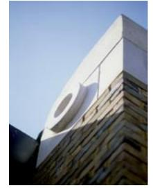
Corner 'acroteria' doubling as ancient horn-images, gutter overflows and brick wall compressors.
