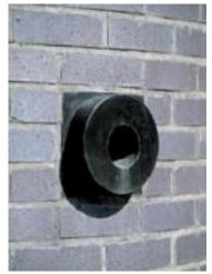
The outlet of the rainwater pipe from the monostyle column was cast in black concrete and then clearlacquered to shine a deep sable.
